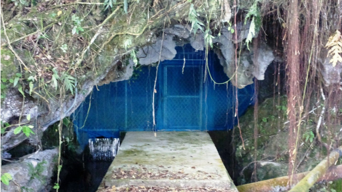
Figure 13. January 2014 photograph of the entrance of Sonson Water Cave showing catchment structures and public access barrier. (Photo by Mike Richardson)
